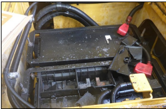
Image 1: Failed battery in Cat 993K front end loader
